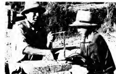
89. Eugenio and aid, making roof tiles.
