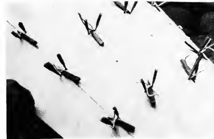
41. Ribs, with strings, pegs and wedges, to form the concave bottom.
